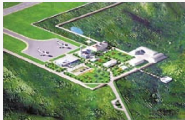
A recent RMB 140 million investment grant by the central government brings total investment of Qianjiang Zhubai Airport to RMB 317 million
