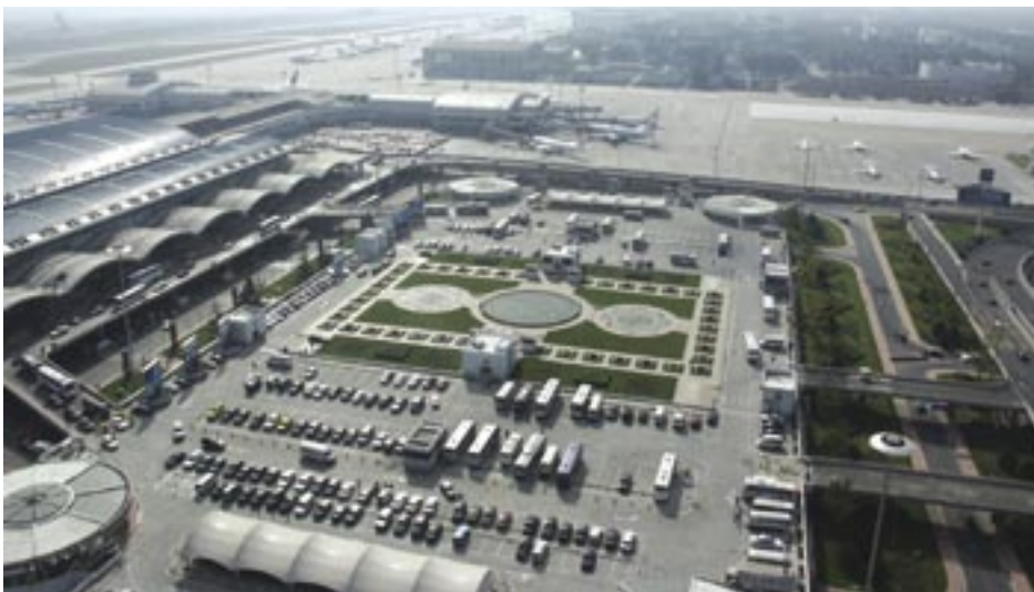
Beijing Capital Airport and China Aviation Oil Group Company finalized a RMB 317 million expansion project to provide increased fueling capabilities to BCIA in late July
