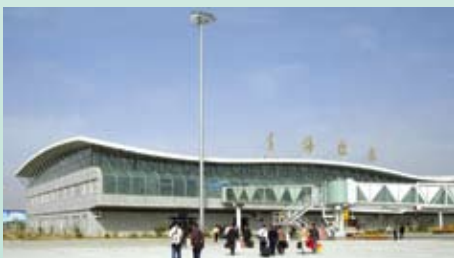
Hailar Airport's newest runway is now ready for action.
