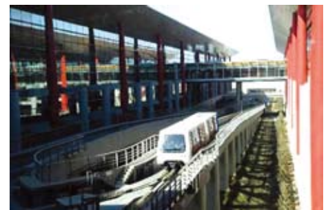
BCIA passengers can access the three sections of T3 via shuttle train.
